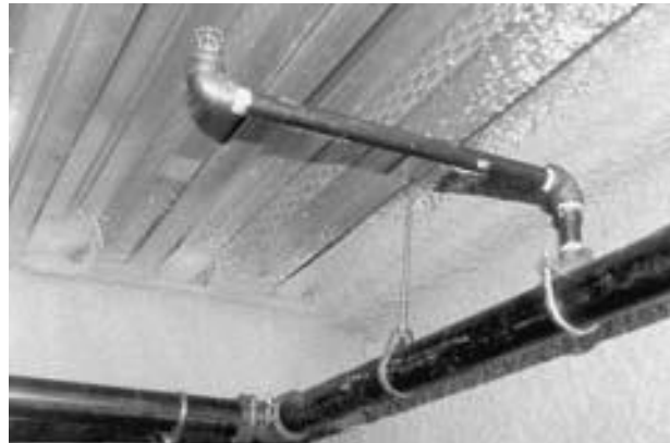
FIGURE A.9.2.3.5 Maximum Length for Unsupported Armover.
