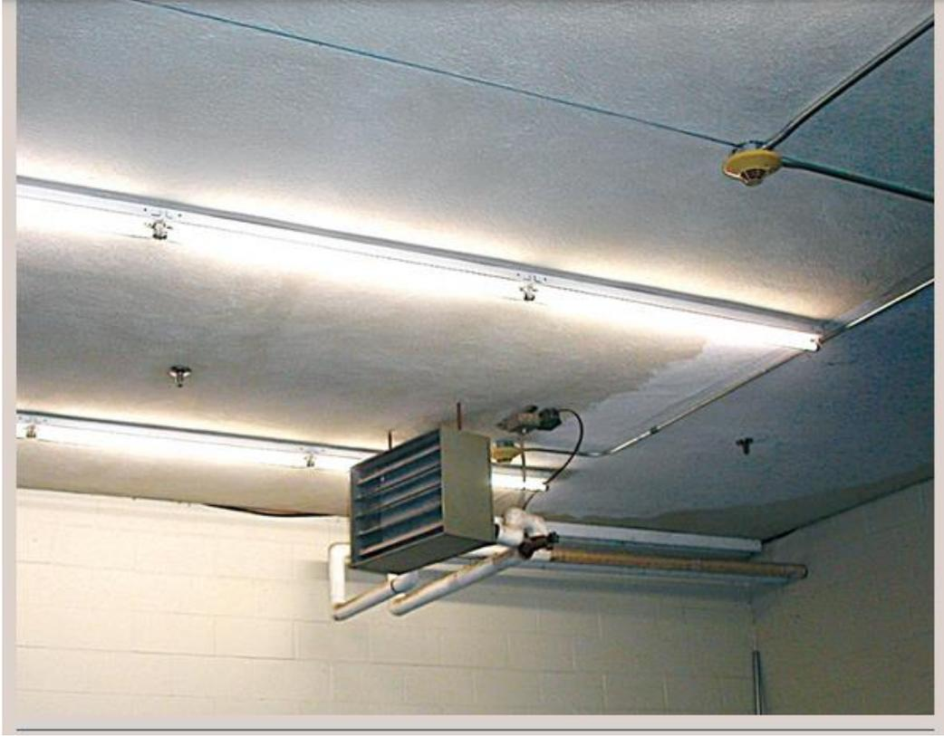
The picture shows two sprinklers installed in the vicinity of a unit heater. The sprinkler in front of the unit heater is required to be a high-temperature sprinkler because it is located within the 7 ft (2.1 m) high-temperature zone established in [Table 8.3.2.5\(a\)](#) and [Figure 8.3.2.5](#). The sprinkler located behind the heating unit is outside the high-temperature zone so it is permitted to be an ordinary-temperature sprinkler.
