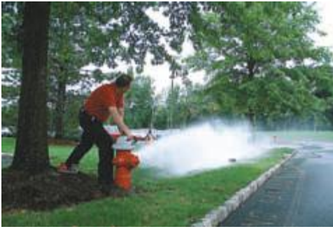
Flushing of Residual Hydrant (left) and Attachment of Test Equipment (right).
