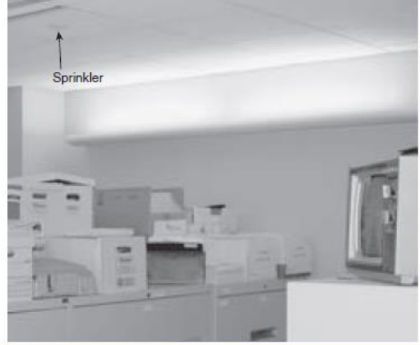
EXHIBIT 8.25 Examples of Storage Room Clearances: (left) Room with Storage Against Wall Extending to Ceiling with Sprinklers and (right) Storage Room with Proper Clearance Below Sprinklers.
