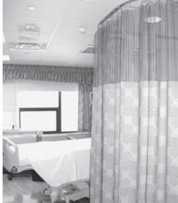
EXHIBIT 8.24 Example of Health Care Privacy Curtain with Sprinklers: (left) Piece of Mesh Used for Curtains and (right) Mesh Curtain Installed. (Courtesy of Tana-TEX, Inc.)
