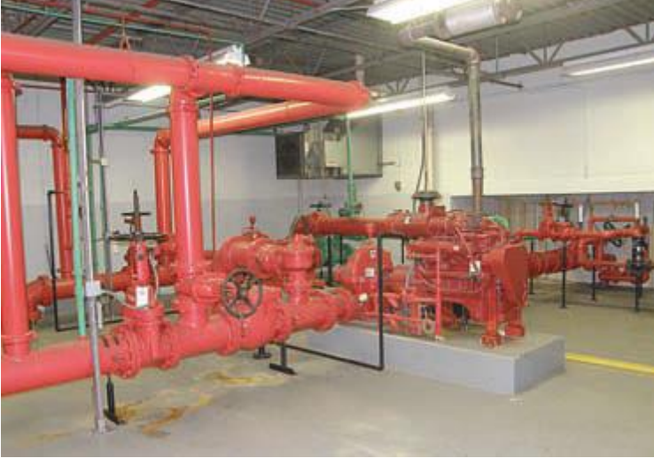
Grooved Fittings and Couplings and Flanged Fittings.
