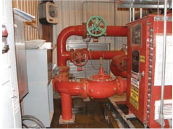
EXHIBIT II.4.15 Low Suction Throttling Valve. (Courtesy of Aon Fire Protection Engineering)
