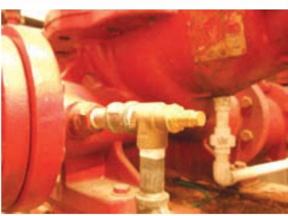
EXHIBIT II.4.7 Circulation (Casing) Relief Valve.
