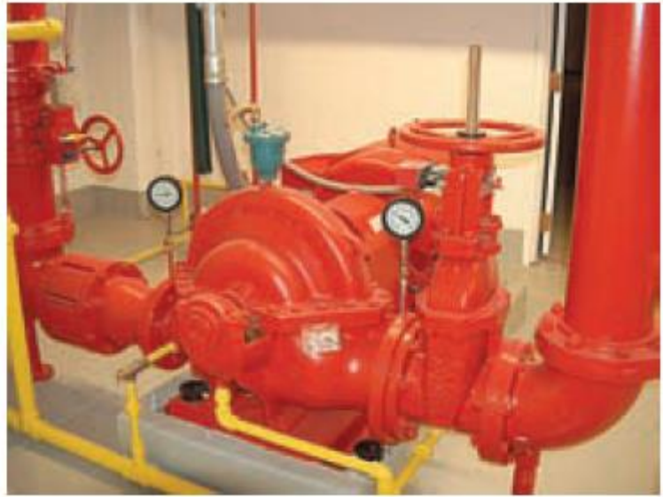
EXHIBIT II.6.3 Single-Stage Axial (Horizontal) Split-Case-Type Centrifugal Pump. (Courtesy of Schirmer Engineering Corp.)
