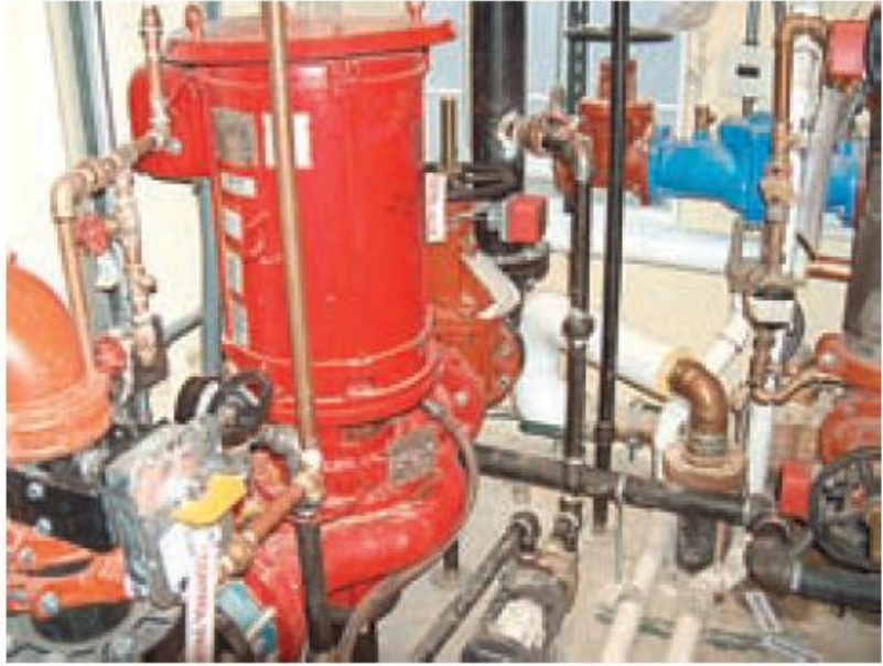
EXHIBIT II.6.4 Radial (Vertical) Split-Case-Type Centrifugal Pump. (Courtesy of Schirmer Engineering Corp.)
