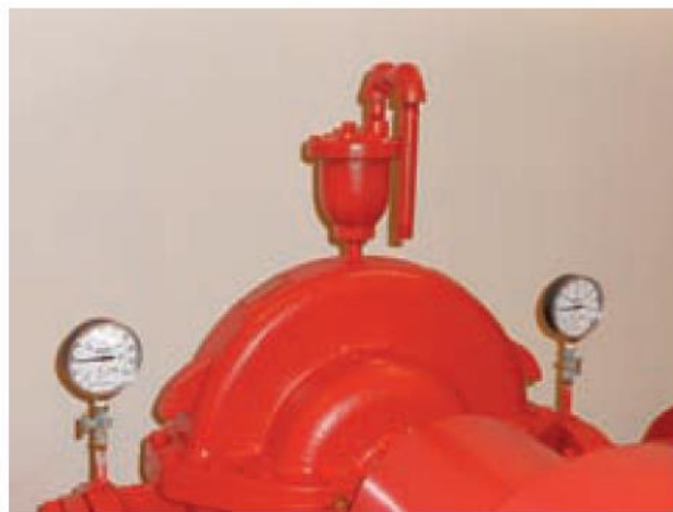
EXHIBIT II.6.11 Automatic Air Release Valve. (Courtesy of Global Vision Inc.)
