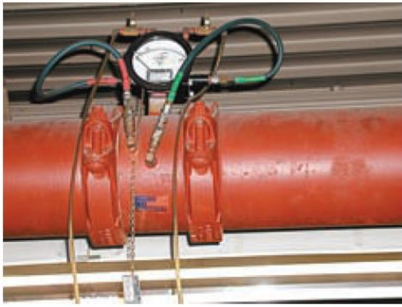
EXHIBIT II.14.7 Determining Flow Using a Flowmeter. (Courtesy of Underwood Fire Equipment, Inc.)
