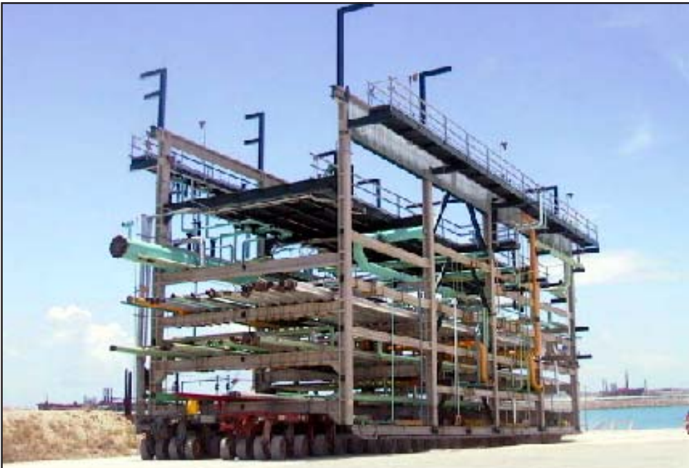
Figure 7.1-11 KAMAG Self-Propelled Transporters Hauling Module
