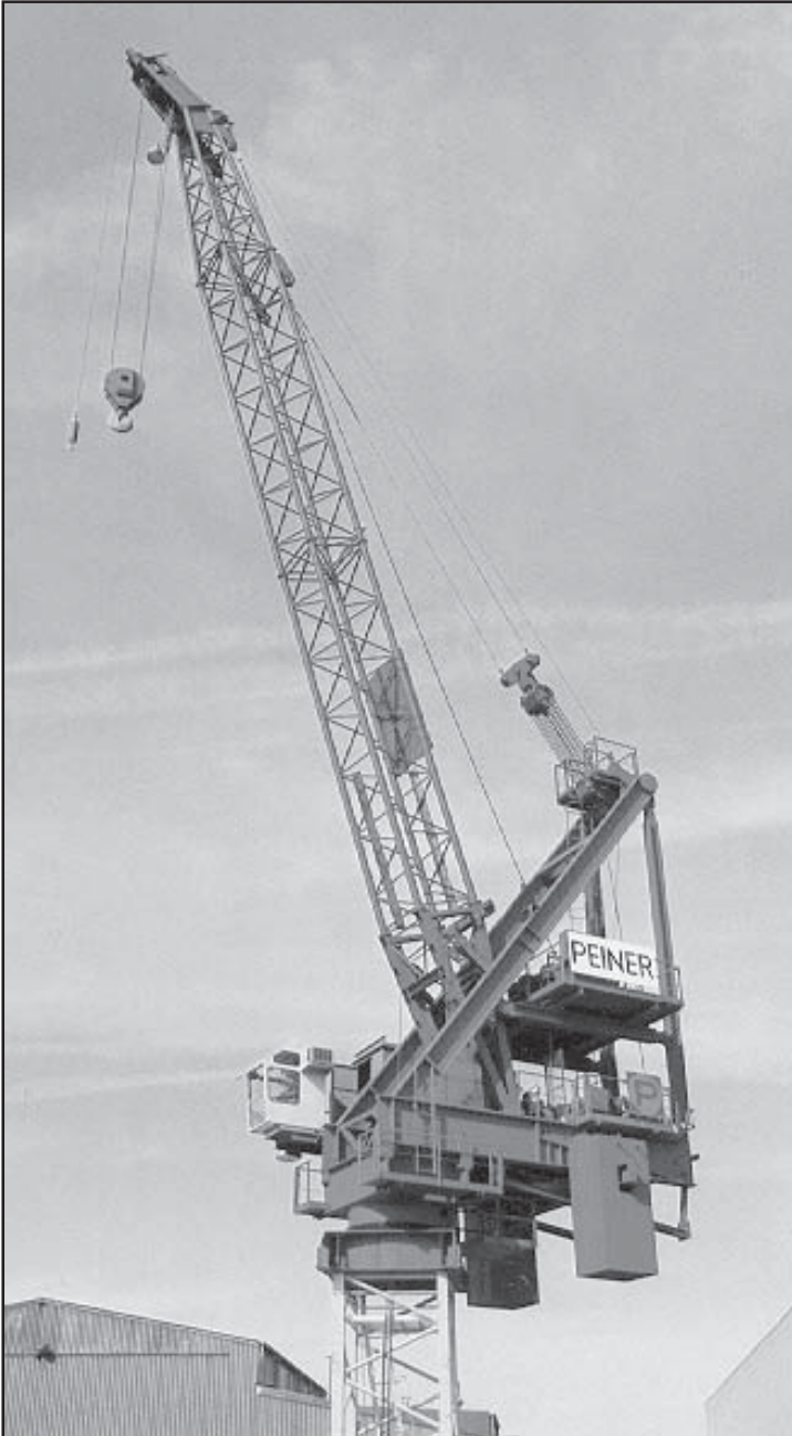
Figure 3.4-2 Luffing Jib Tower Crane
