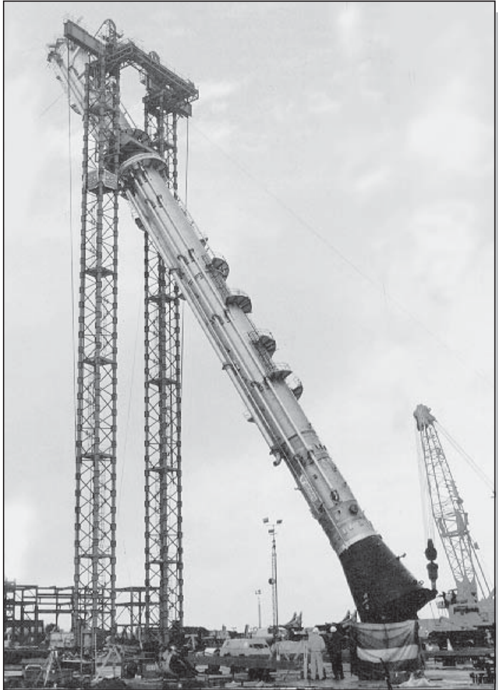
Figure 5.7-2 Gallows Pole Arrangement
