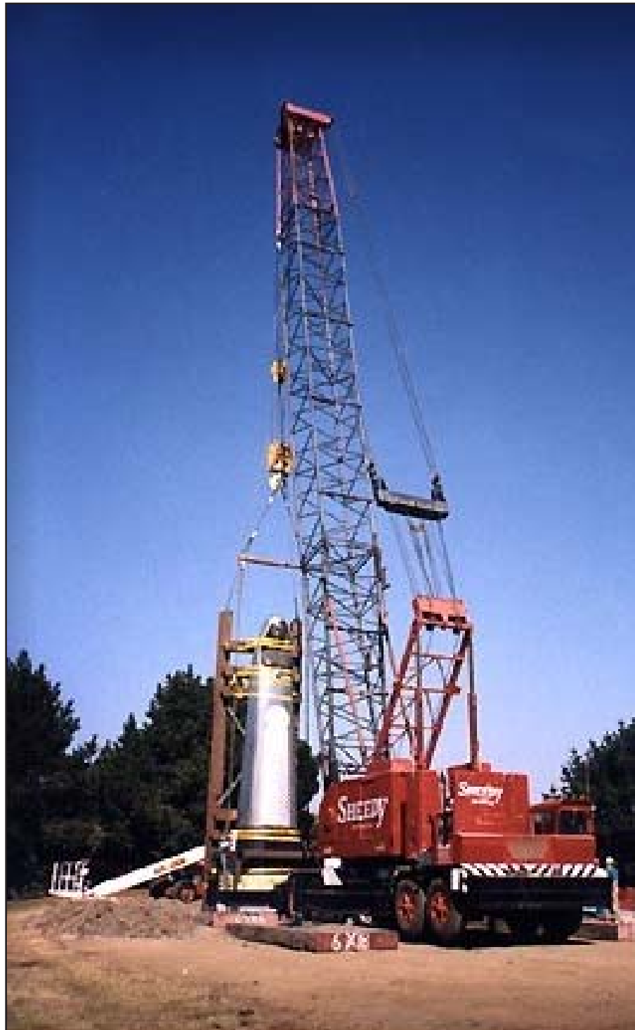
Figure 3.5-8 Lattice Boom Truck Crane
