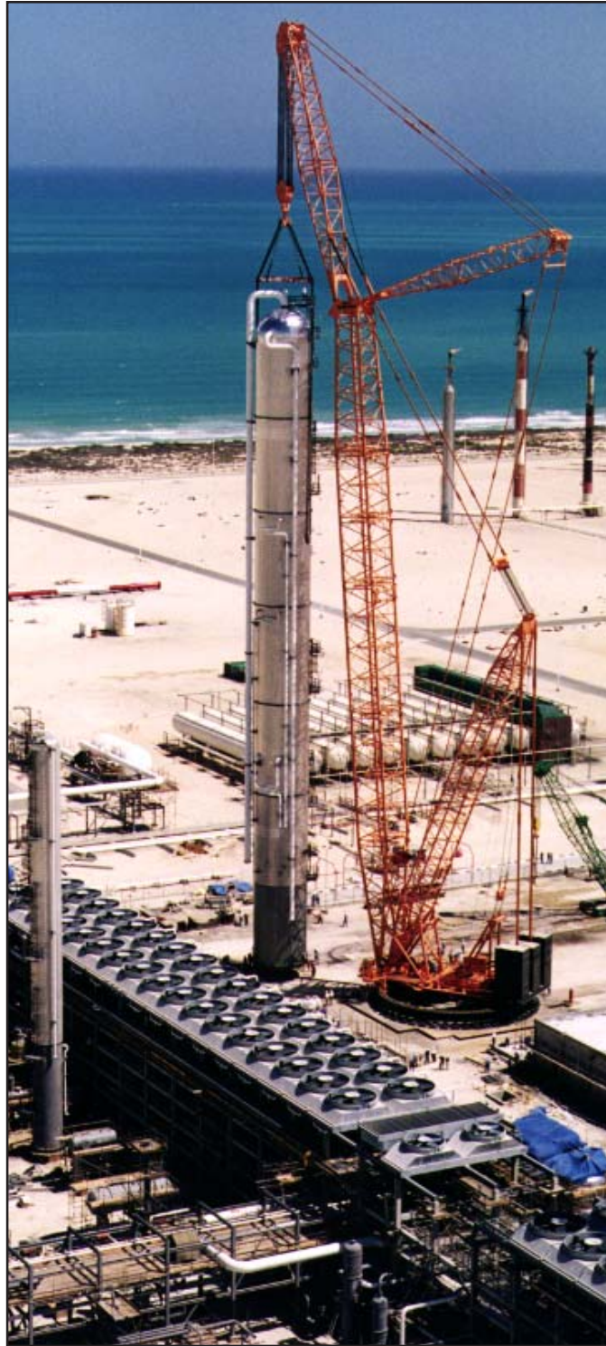
Figure 3.6-2 Ringer Attachment
