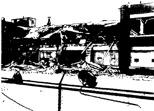
Figure 38 Damage to this laboratory building resulted from a flash fire and explosion following the rupturing of a sampling container.
