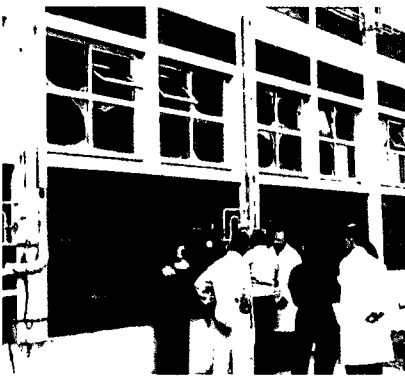
Figure 50a Damage caused by flexible hose rupture.
