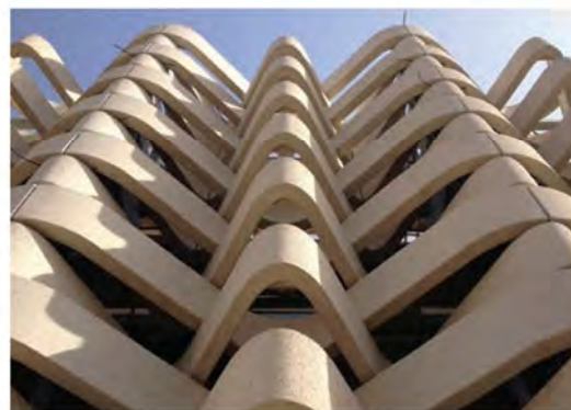
Cooling Tower, Doha
