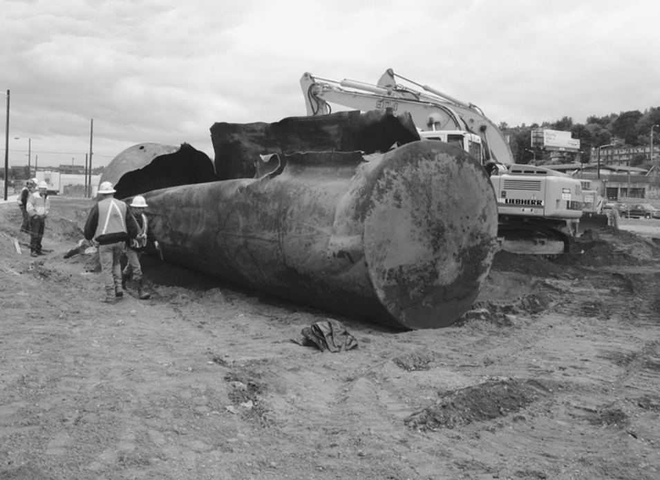
Cleanup of a brownfield site in Oregon contaminated with volatile organic compounds. Brownfields are abandoned or little-used industrial or commercial sites contaminated with toxic chemicals or other hazardous substances. (Environmental Protection Agency)
