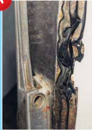
Defective refrigerator door seals should be replaced
