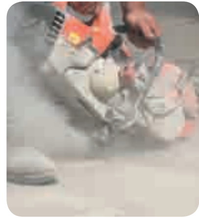
Construction worker using portable power tool
