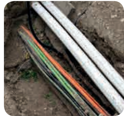
A shallow excavation revealing a collection of buried services
