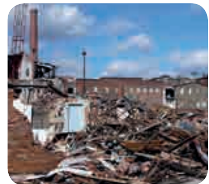
Temporary works include demolition
