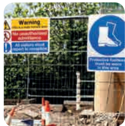
Perimeter fencing with safety signs
