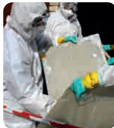
Removal and bagging of ACM
