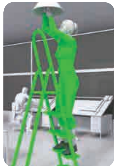
Correct use of a stepladder for a brief task where two hands need to be free. (Source: INDG455 Safe use of ladders and stepladders - A brief guide, HSE, 2014 - www.hse.gov.uk/pubns/indg455.pdf )
