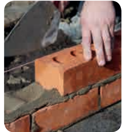
Suitable PPE should be provided for bricklayers
