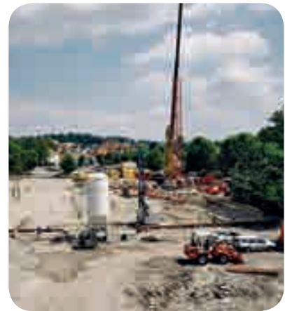
Cement is used extensively in the construction industry
