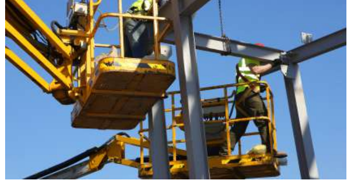
Steel workers use MEWPs to gain access to a structural steel that is being lifted into place. Note the use of full body harness despite being in an enclosed cradle.
