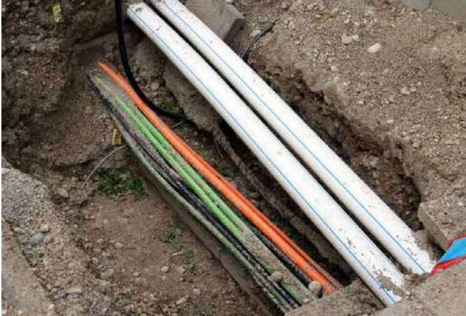
A shallow excavation revealing a collection of buried services
