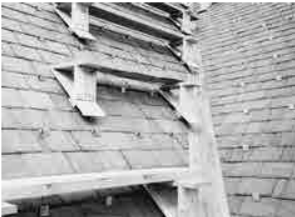
FIGURE 8.37 Example of roof bracket scaffolds
