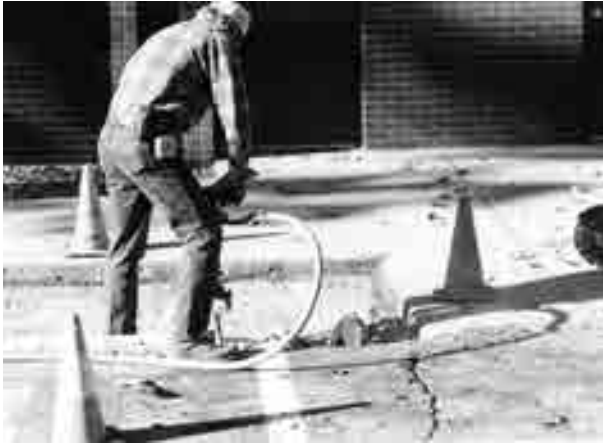
FIGURE 11.11 Worker using a pneumatic jack hammer
