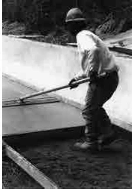
FIGURE 7.13 Construction worker using a bull float
