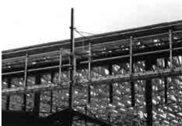
FIGURE 8.38 Pump jack scaffold
