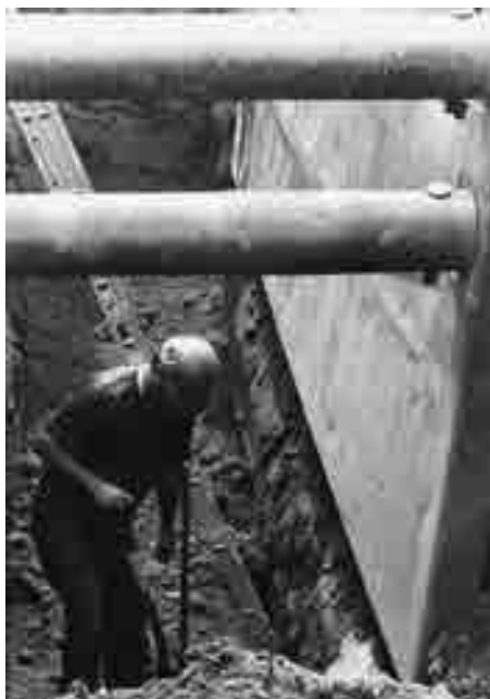
FIGURE 7.39 Worker using a trench box as a shield with a ladder for egress
