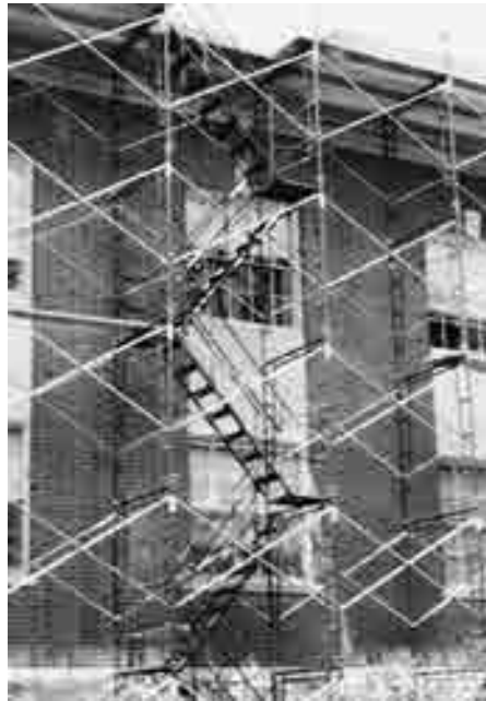
FIGURE 8.35 Built-in scaffold access ladders
