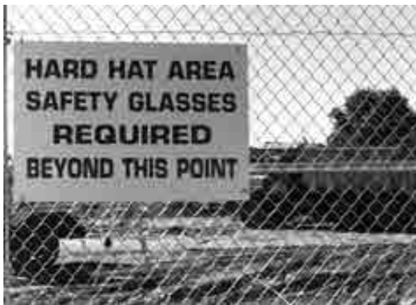
FIGURE 8.40 Warning sign for site requirements
