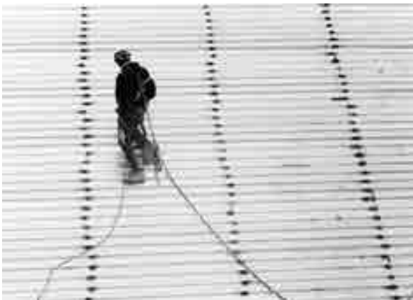
FIGURE 11.16 Roofer working on slanted surface
