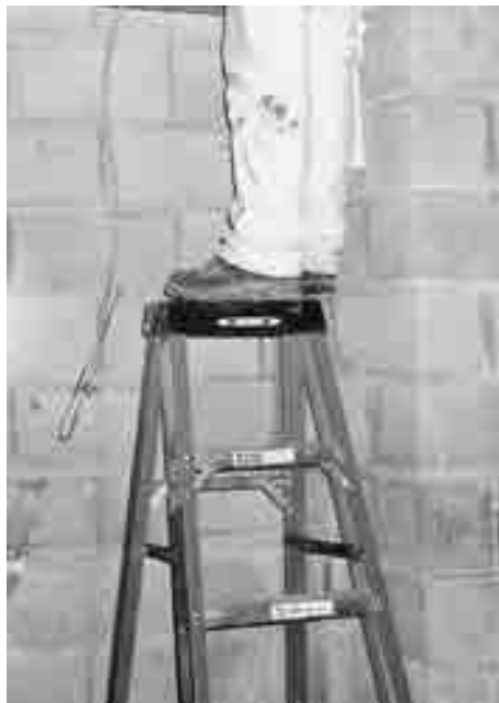
FIGURE 8.4 Unsafe use of a stepladder by standing on top step
