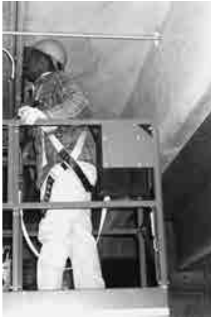
FIGURE 7.48 Personal fall protection system
