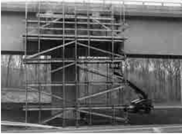
FIGURE 8.36 Example of a pole scaffold
