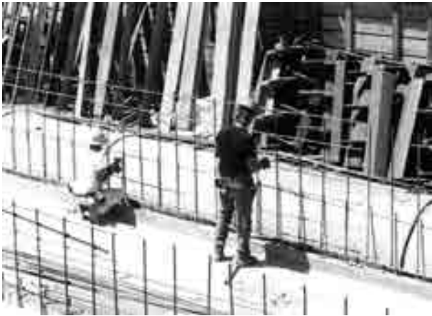
FIGURE 11.14 Construction workers tying rebar
