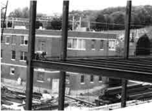
FIGURE 11.13 Steel worker bolting a steel member into place
