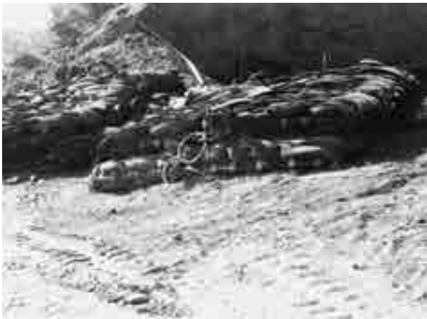
FIGURE 7.40 Example of blasting mats
