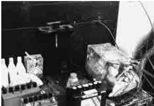
FIGURE 7.7 Poorly designed battery charging area
