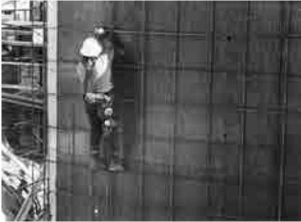
FIGURE 1.1 Ironworker tying rebar on a lattice
