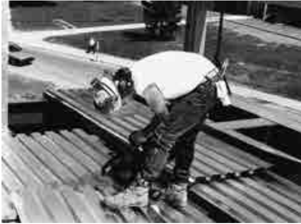
FIGURE 7.43 Worker using a chop saw with eye and hearing protection
