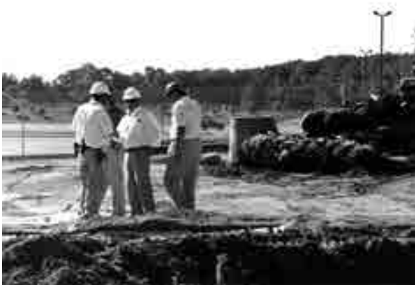
FIGURE 18.4 The contractor's presence and communication demonstrate his or her commitment to a safe and productive construction site
