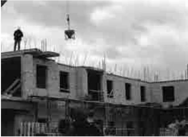
FIGURE 7.11 Concrete bucket in use on construction site
