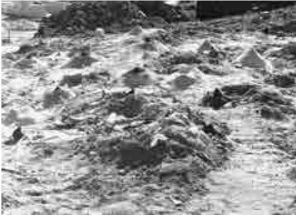
FIGURE 7.42 Drilled blasting area ready for loading
