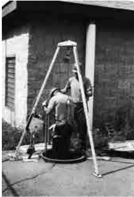
FIGURE 7.18 Confined space worker retrieval system with attendant
