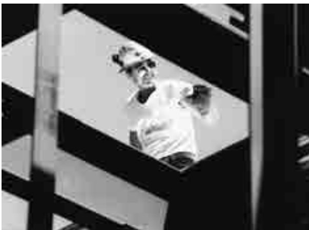
FIGURE 9.2 The construction site is constantly changing
