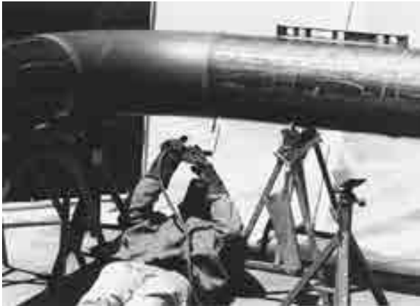
FIGURE 10.4 Welding is a classic generator of ultraviolet rays
