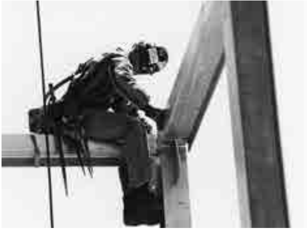
FIGURE 8.46 Steel worker trying to align the members prior to bolting
