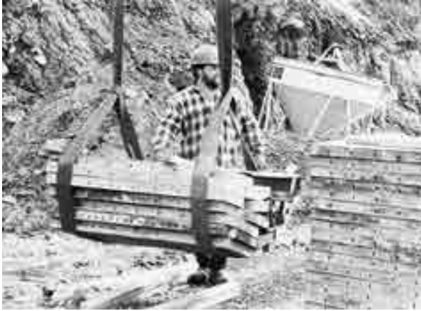
FIGURE 8.27 Web sling being used on construction site
