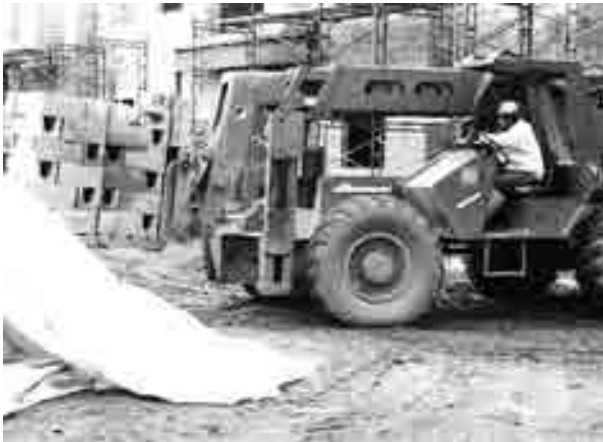
FIGURE 11.25 Palletized concrete blocks being moved by a pallet truck
