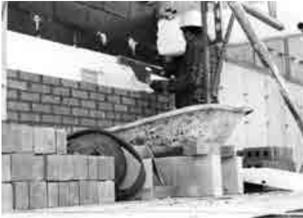
FIGURE 11.12 Typical bricklayer work and work area
