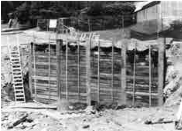
FIGURE 7.38 A timber shored wall of an excavation
