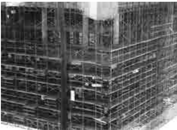
FIGURE 8.32 A large scaffold system encompassing an entire building
