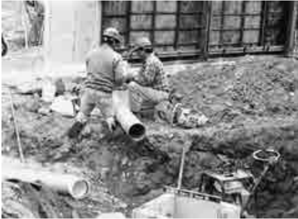
FIGURE 2.1 Typical construction workers laying pipe
