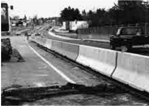
FIGURE 7.5 The use of jersey barriers as barricades
