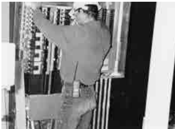
FIGURE 7.24 Electrician with adequate working clearance
