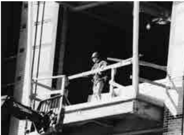
FIGURE 7.44 Worker with personal fall protection in a hoist area
