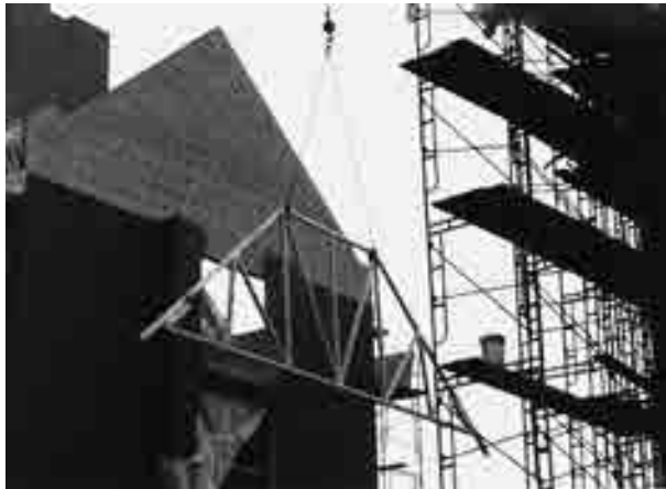
FIGURE 8.24 Example of wire rope slings being used
