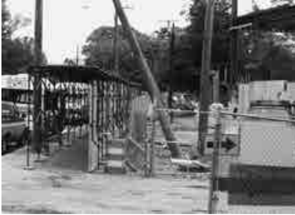
FIGURE 7.45 Canopy for overhead protection
