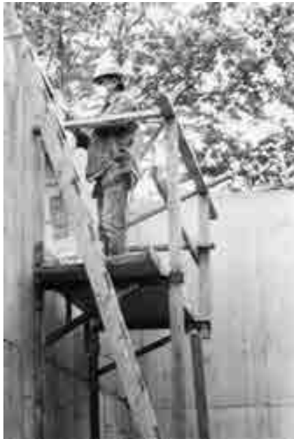
FIGURE 8.33 A full planked scaffold with guardrails
