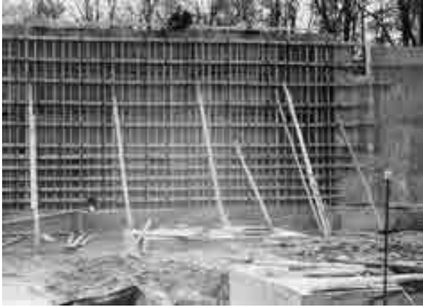
FIGURE 7.14 Formwork for cast-in-place concrete
