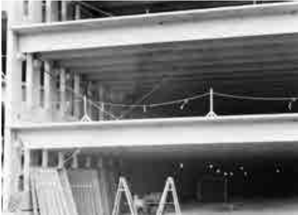
FIGURE 8.19 Example of construction of a precast parking garage
