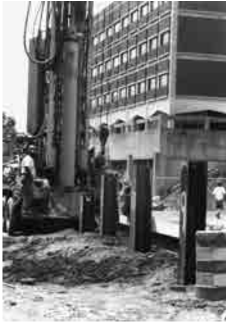
FIGURE 8.12 Example of piles being driven
