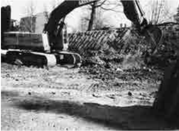
FIGURE 7.37 Example of sloping and excavation
