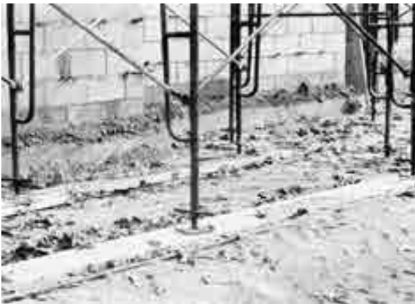
FIGURE 8.34 Scaffold legs and base plates supported on mud sills
