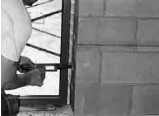
FIGURE 8.15 Powder-actuated tool being used to drive fasteners into masonry wall
