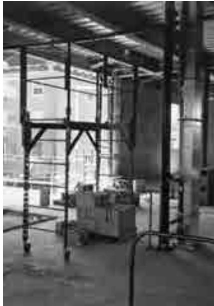
FIGURE 8.39 Example of a mobile scaffold
