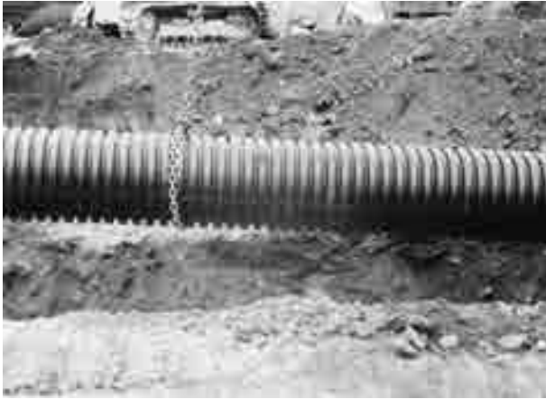
FIGURE 8.23 Chain using a choker hitch for lifting
