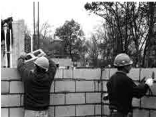
FIGURE 11.8 Mason laying block above shoulder height
