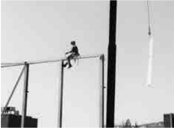
FIGURE 8.44 A steel worker's precarious perch
