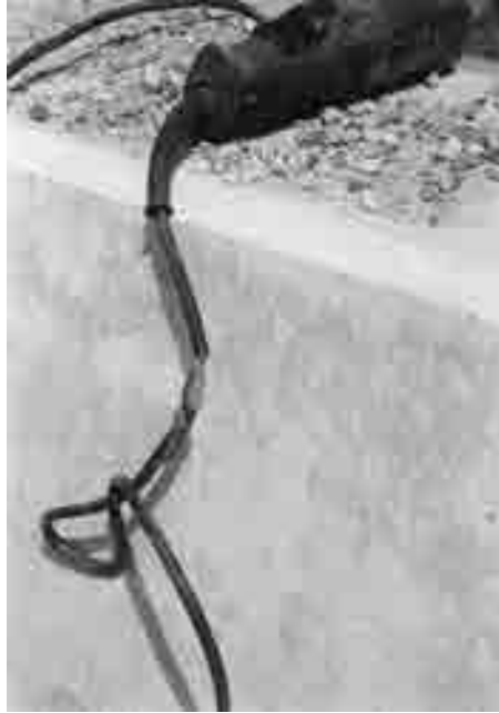
FIGURE 8.17 Damaged electrical power tool on a construction site which should be removed from service
