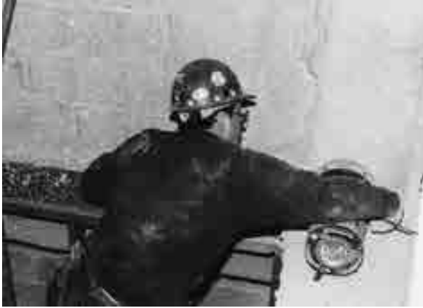
FIGURE 8.21 Construction worker using a laser for leveling operations
