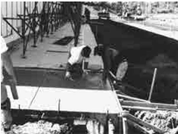
FIGURE 9.1 Today's construction site
