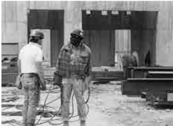
FIGURE 1.5 Ironworkers preparing to rig
