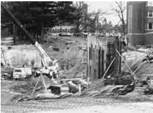
FIGURE 1.7 The always changing construction site
