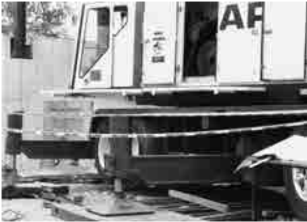
FIGURE 7.20 Crane with outrigger deployed and warning barriers
