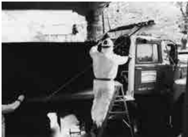
FIGURE 7.57 Trained workers doing hazardous waste work
