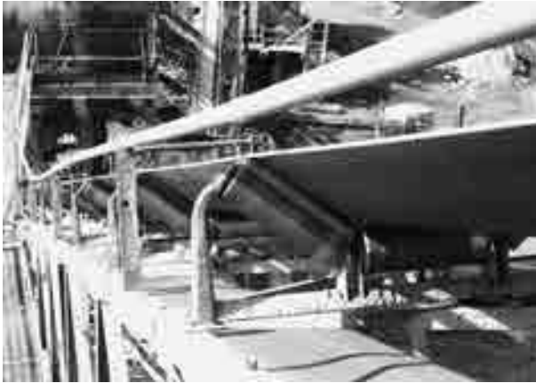
FIGURE 7.19 Example of conveyor hazards with some guarding
