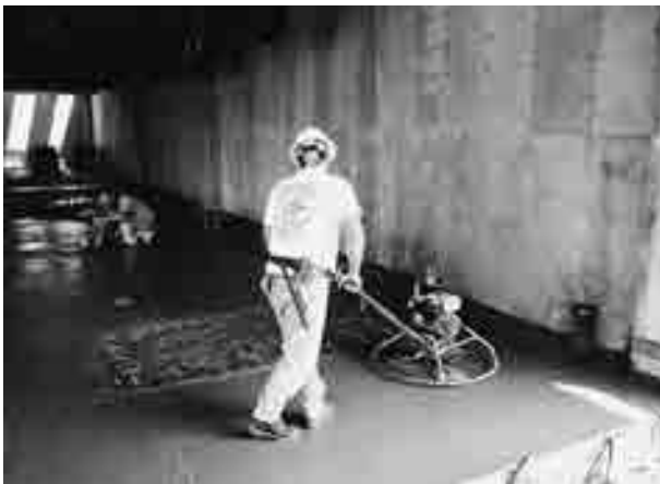
FIGURE 7.12 Worker using a powered trowel
