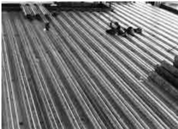
FIGURE 8.45 Flooring installed during steel erection
