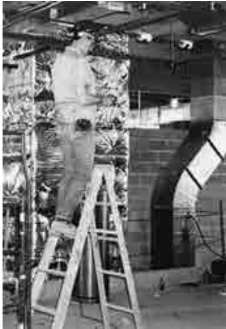
FIGURE 8.1 The safe use of a stepladder is standing no higher than the second step from the top
