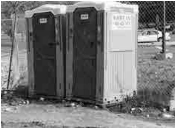
FIGURE 8.48 Typical toilets found on construction jobsites
