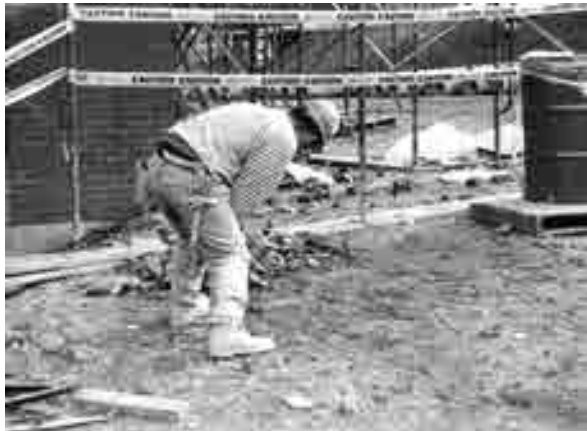
FIGURE 11.4 The movement of a worker's feet is especially critical during shoveling
