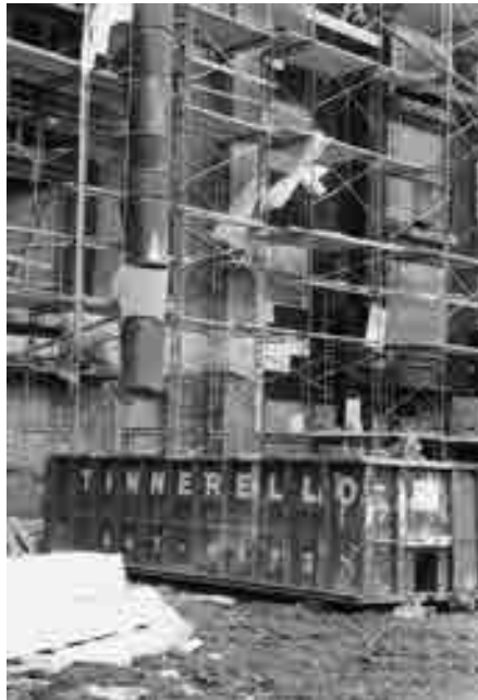
FIGURE 7.23 Enclosed disposal chute on exterior of building
