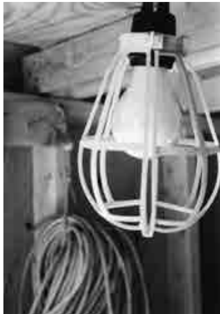
FIGURE 7.30 Protected temporary lighting
