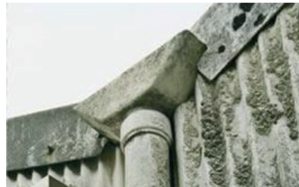
Asbestos cement down-pipe hopper and sheeting
