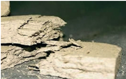
Asbestos insulation board (AIB)
