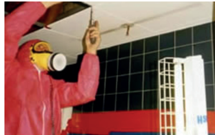
Unscrewing AIB ceiling Boards
