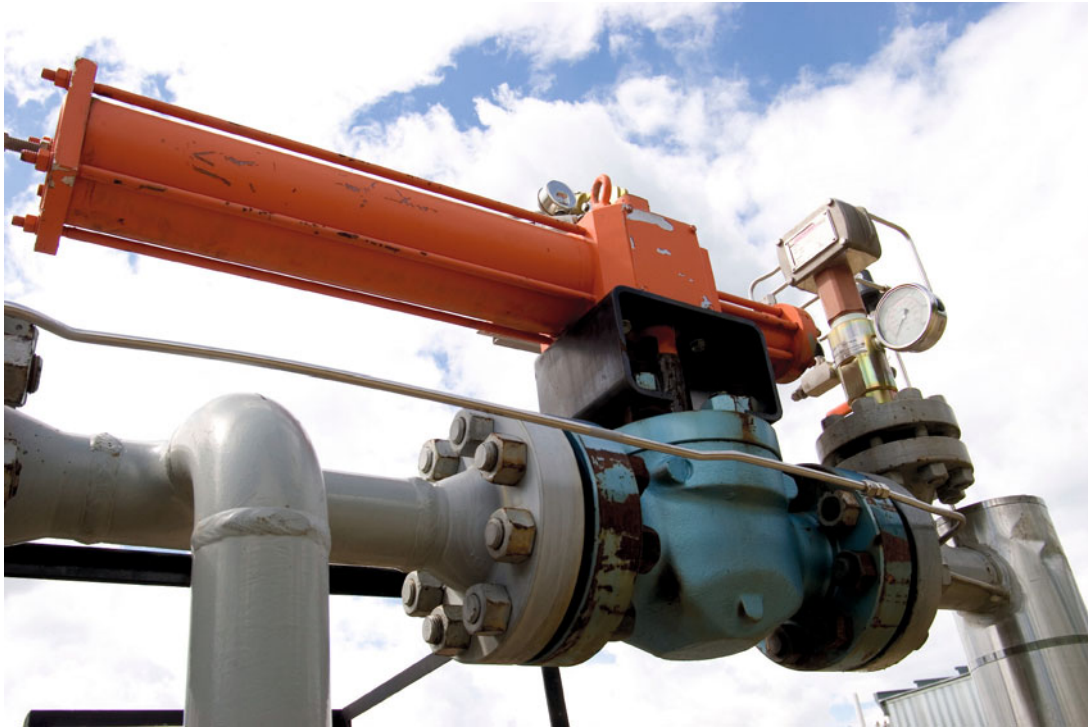
Figure 9.3 Emergency shutdown valve Source: iStock.
