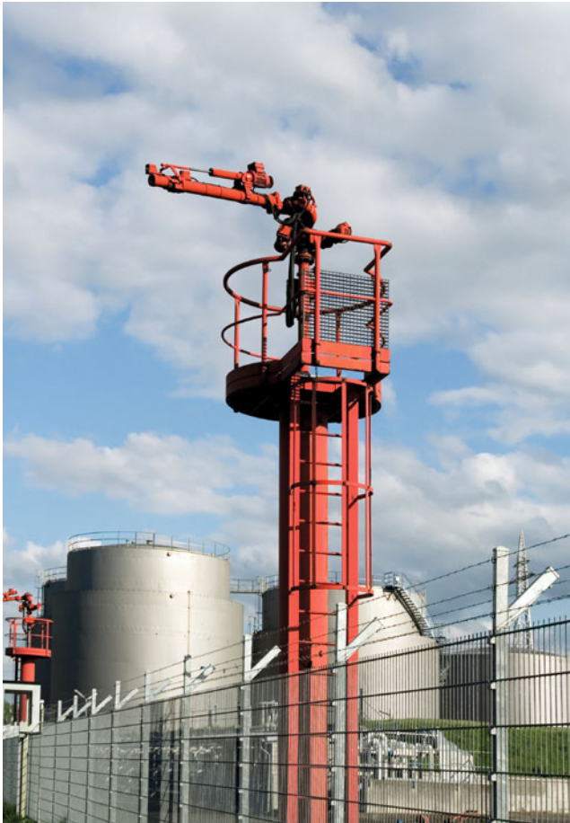
Figure 17.13 Fixed point fire-fighting cannon Source: iStock.
