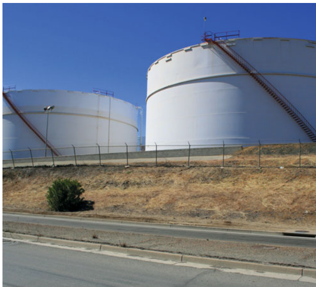
Figure 14.5 Bunded storage tanks
