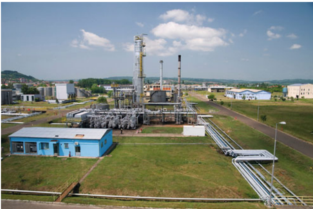
Figure 11.5 U-shaped configuration in pipework Source: iStock.
