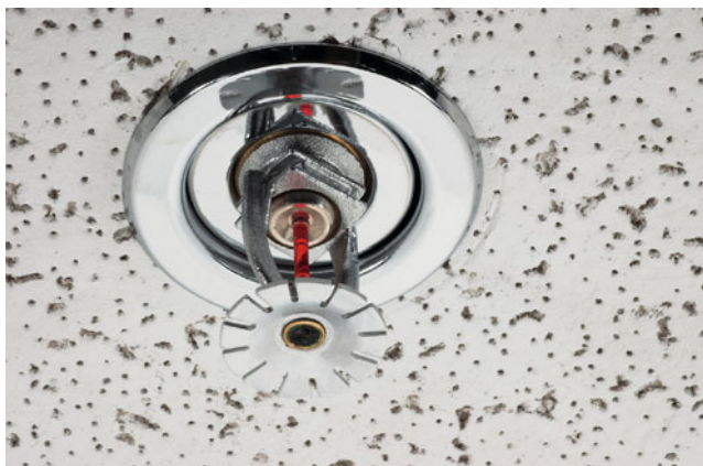
Figure 17.4 Sprinkler head Source: iStock.
