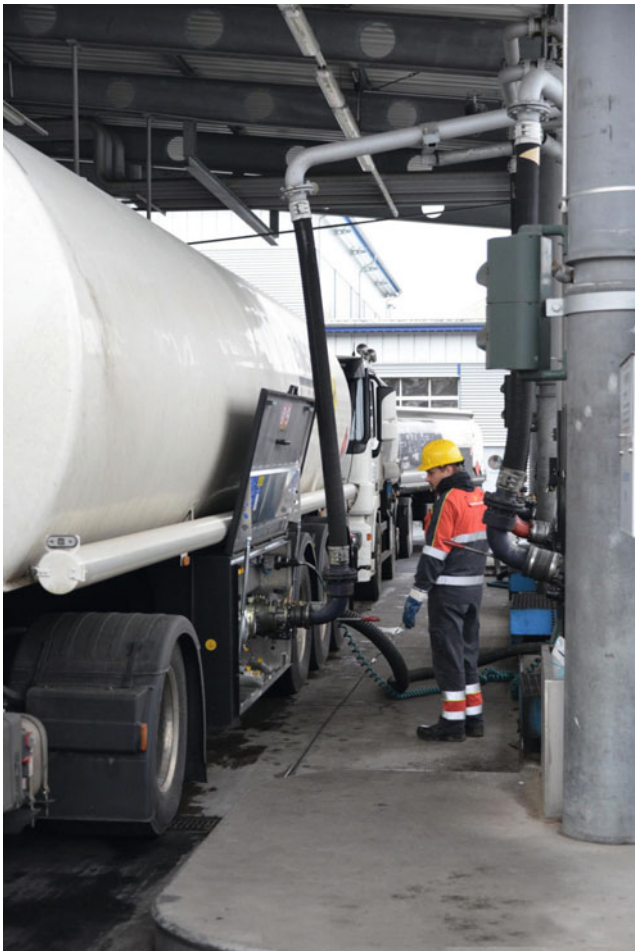
Figure 14.7 Bottom loading of tanker Source: Loadtec Engineered Systems Ltd.
