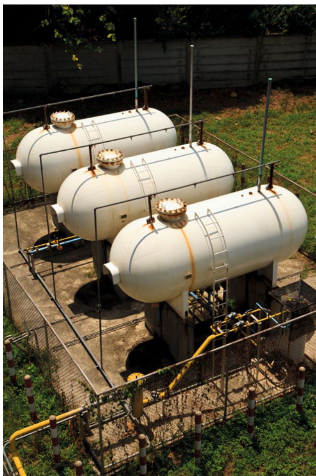
Figure 14.10 Cylindrical storage tanks Source: Dreamstime.
