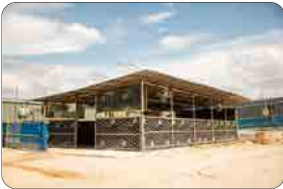
Figure 6: Shaded rest point for workers at a construction site equipped with rotating fans and water coolers. Encourage workers to sponge or rinse themselves with water e.g. during breaks. Body cooling is important especially on days when the weather is hot.
