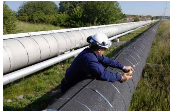
Inspection of the integrity of a pipeline
