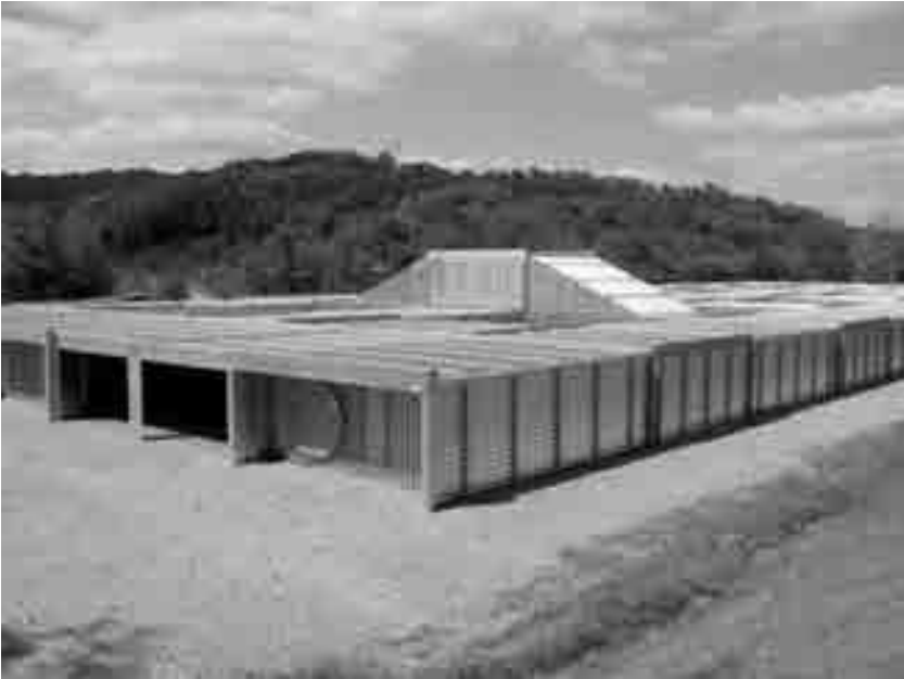
Figure 12.2 A simulated underground mine has been constructed at West Virginia University.
