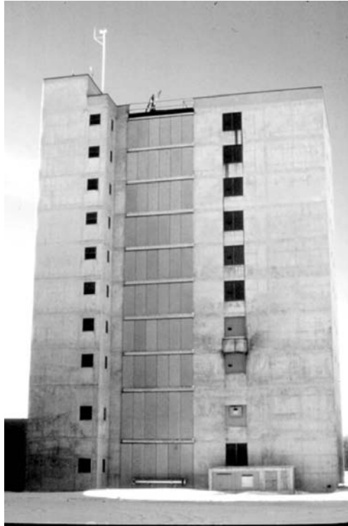
Figure 9.8 The ten-storey experimental tower at the National Research Council Canada for smoke spread and smoke control studies (photo by author, reproduced by permission of the National Research Council Canada).
