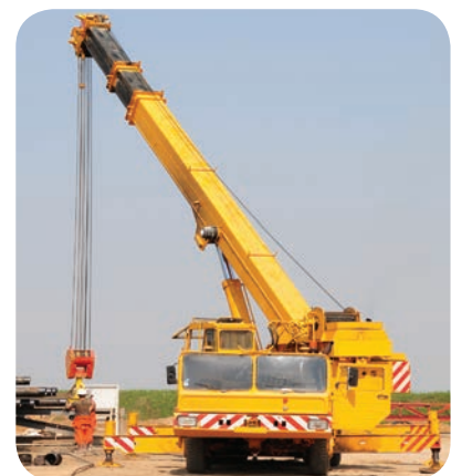
A crane driver must have a full view of the working area
