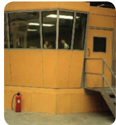
A noise refuge and control room Source: L108 Controlling noise at work (2nd ed.), HSE, 2005 ( www.hse.gov.uk/pubns/priced/l108.pdf )
