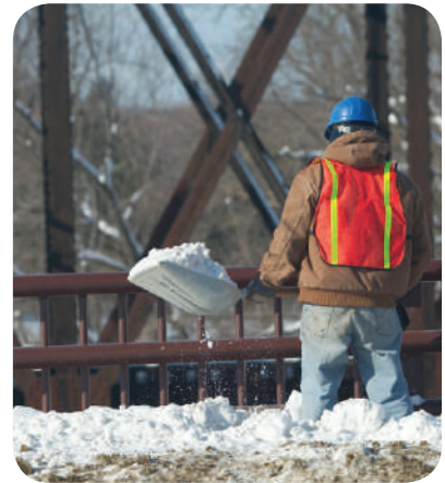
Restrict work during the coldest periods
