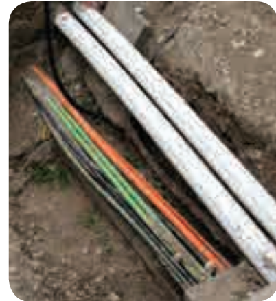
Excavation close to foundations
