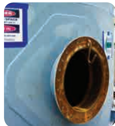
Working in a confined space is a high-risk activity
