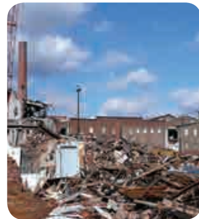
Damage from a dust explosion
