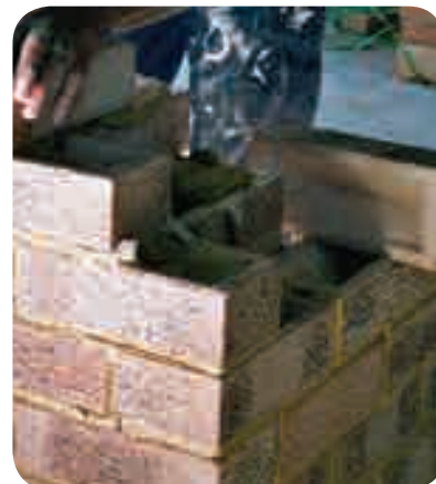
Clay bricks in use on a construction site
