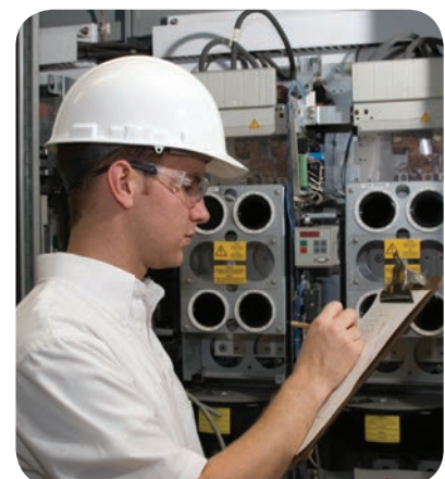
Planned preventive maintenance in progress
