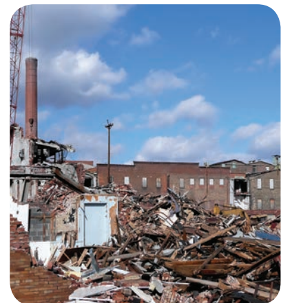
Damage from a dust explosion
