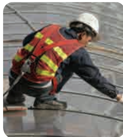
Fragile roof work
