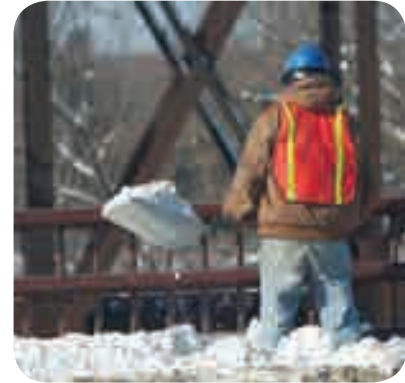
Surface conditions must be considered
