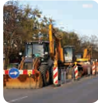
Example of appropriate traffic controls in a workplace
