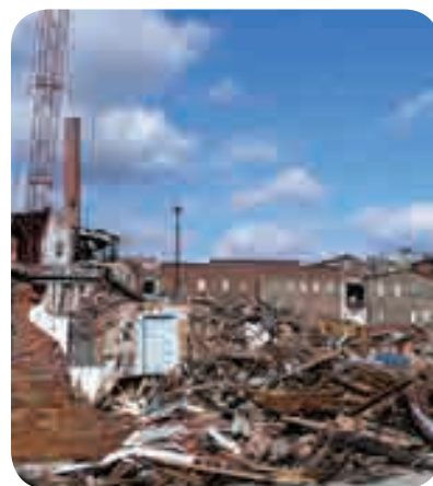
Demolition in progress
