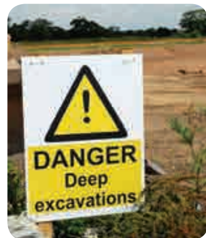
Excavations can cause fatal accidents
