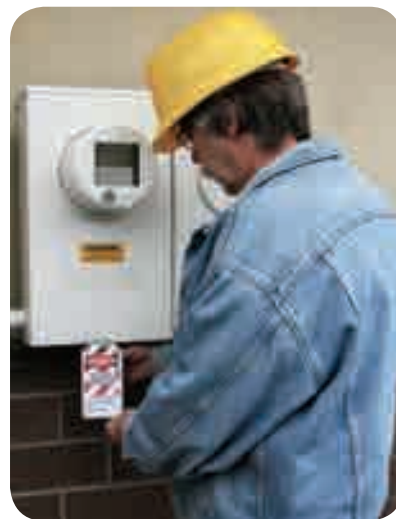
Disconnection of equipment
