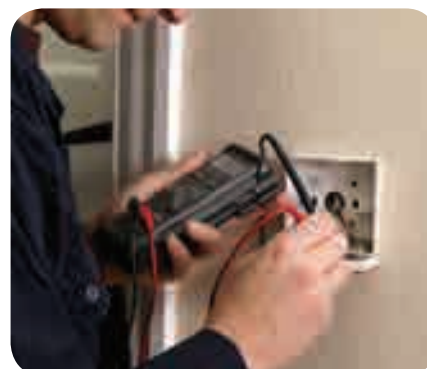
Inspection by a competent person
