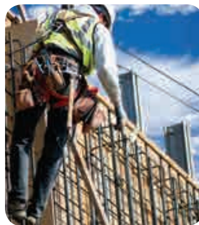
Worker using fall-arrest equipment - note the full body harness with lanyard attached at the back
