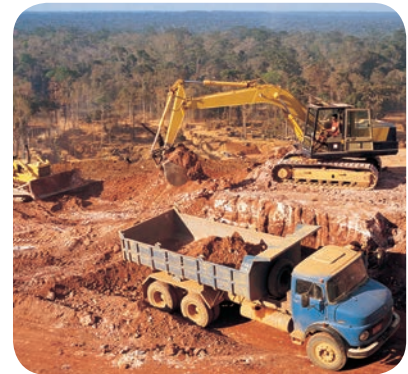
An 'unprepared' route for vehicle operation
