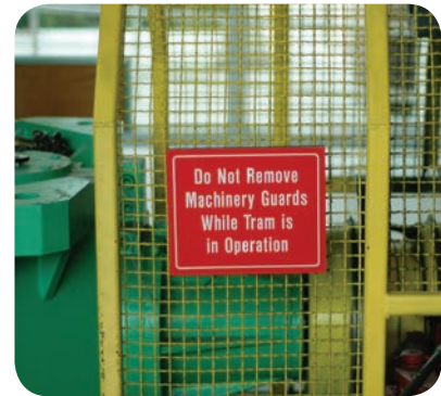
Adequate guarding for machinery with moving parts
