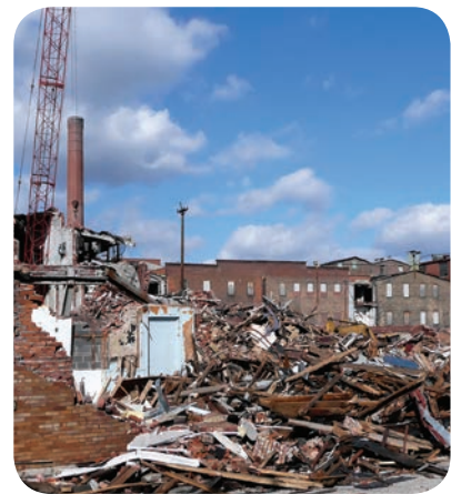
Demolition in progress
