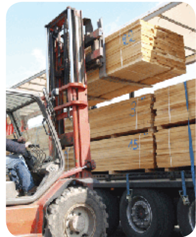
Many accidents occur during loading and unloading of vehicles
