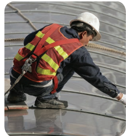
Fragile roof work
