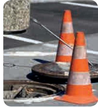
Entry into a sewer - confined space entry
