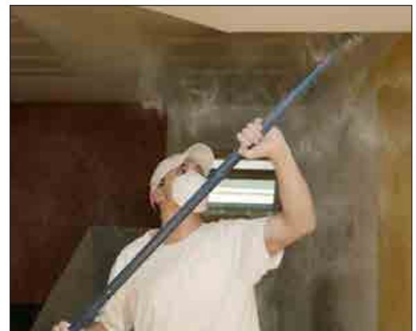
Use handle extensions with auto-feed screw guns, sanding blocks, or taping tools.
