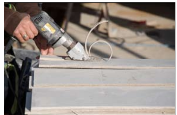
Cutting fibre-cement board with a hand-held shear
