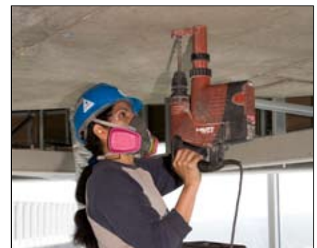
Drilling using a dust cap
