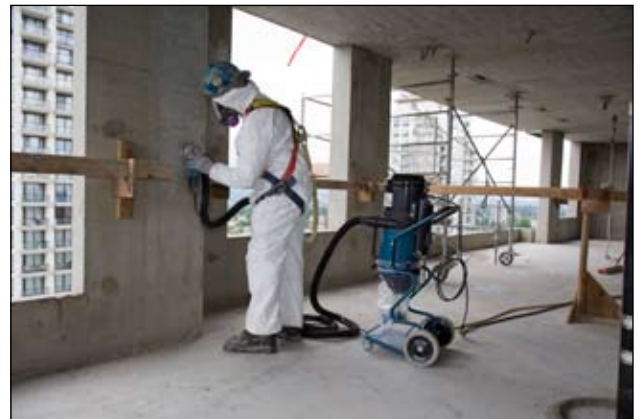
Wall grinding with LEV
