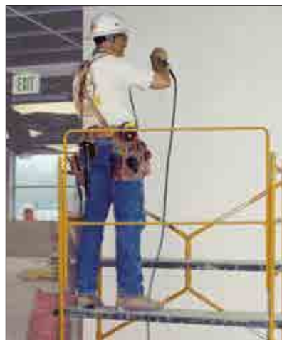
Work from scaffolding.
