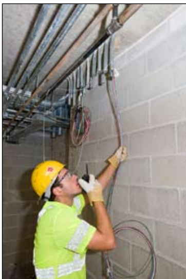
Coordinating the effort makes pulling wire easier.
