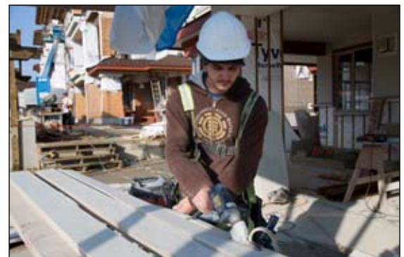
Worker cutting fibre-cement board outdoors, with a hand-held shear
