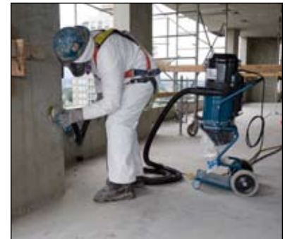
Worker grinding concrete using local exhaust ventilation
