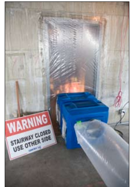
Poly enclosure with HEPA “negative air” unit
