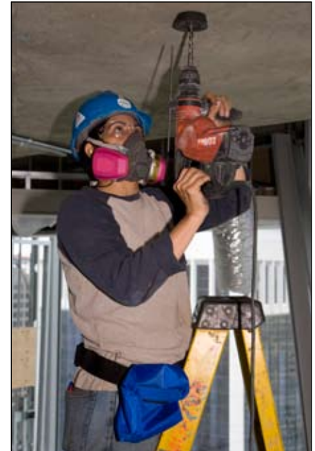
Drilling using a dust cap
