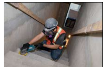
Stair grinding with LEV
