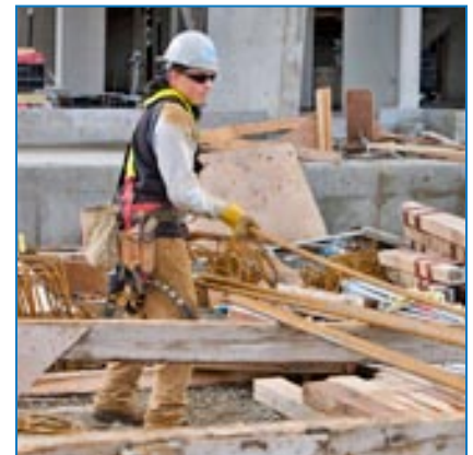
Raise materials to waist height. This reduces forward bending.
