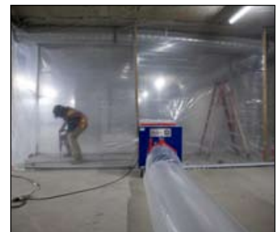
Worker drilling concrete inside an enclosure equipped with a “negative air” unit
