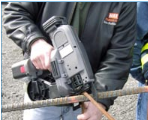
Use a rebar gun. It reduces awkward posture of the wrist when tying rebar.
