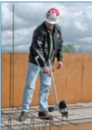
Use a rebar tying machine. It allows workers to tie while standing upright.
