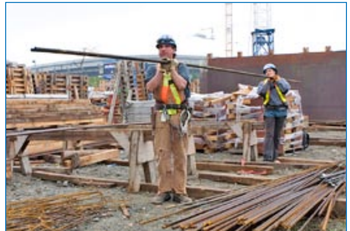
Use the two-person lift procedure. This reduces weight on the shoulder for both workers.
