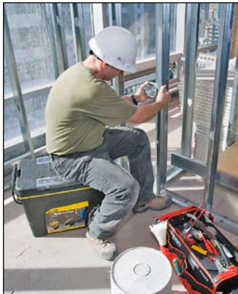
By sitting on a stool, workers avoid bending over at the waist.
