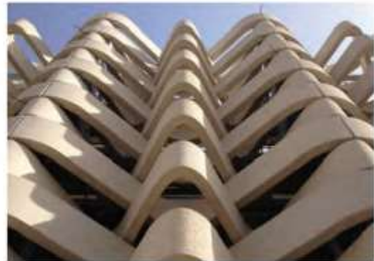
Cooling Tower, Doha
